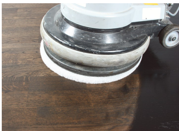
8) Mechanical application of Osmo Polyx® Professional Color Oil
